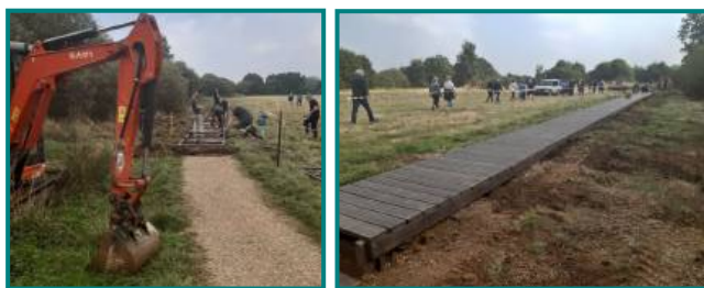
Repairing paths and installing board walks
