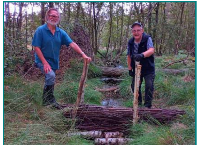
Making a leaky dam.
