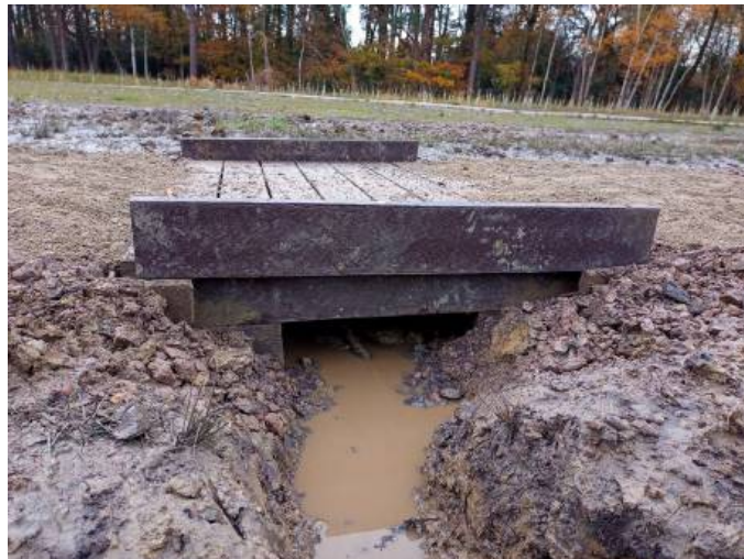
Repair work on Wheatsheaf Common
